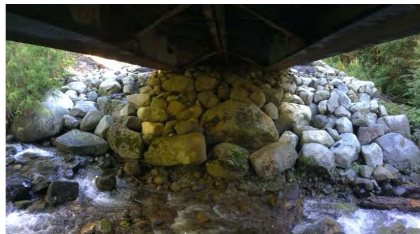
Left Bank Abutment when facing downstream
